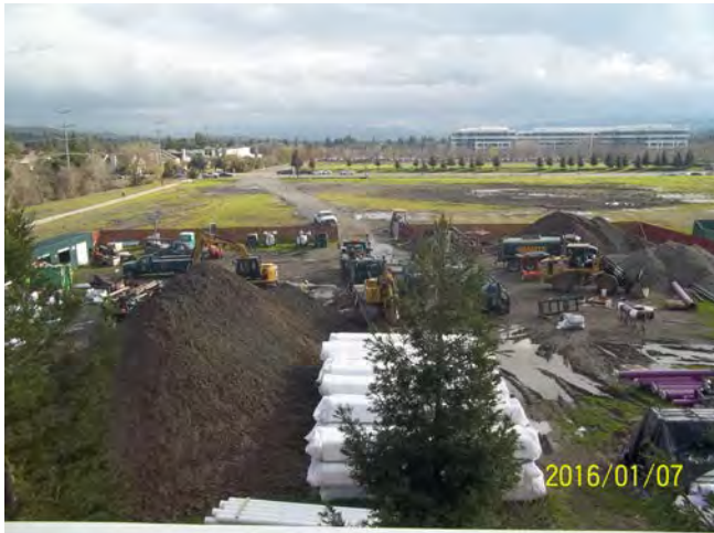
Photo 3: View of the eastern portion of the property, looking south.
