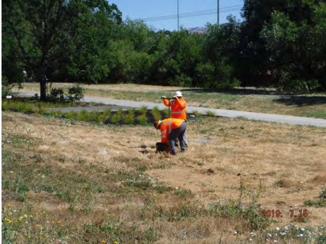
Photo 1: View of drilling boring A-3.
