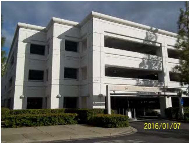
Photo 21: North – Bishop Ranch 3, parking garage (2641 Camino Ramon).
