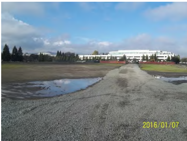
Photo 5: View of gravel access road, looking northwest.
