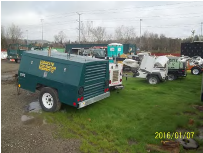
Photo 9: View of typical equipment utilized by Granite Construction.
