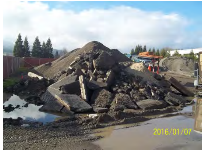
Photo 8: View of asphalt and gravel piles utilized by Granite Construction.
