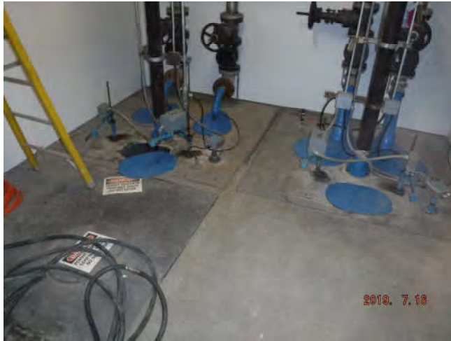
Photo 19: View of two rainwater sumps.
