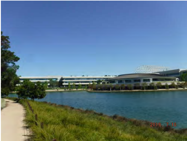
Photo 3: View of the West Lake and West Wing, looking north.
