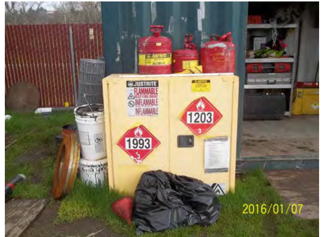
Photo 14: View of typical flammable material storage.
