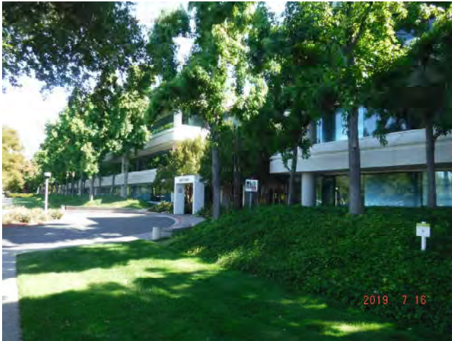
Photo 1: View of the North Wing, looking northeast.
