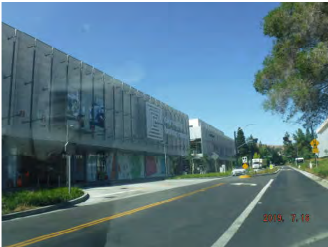
Photo 27: View of the south adjacent sites, looking southwest.
