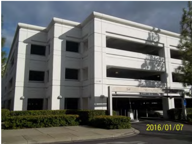
Photo 21: North – Bishop Ranch 3, parking garage (2641 Camino Ramon).
