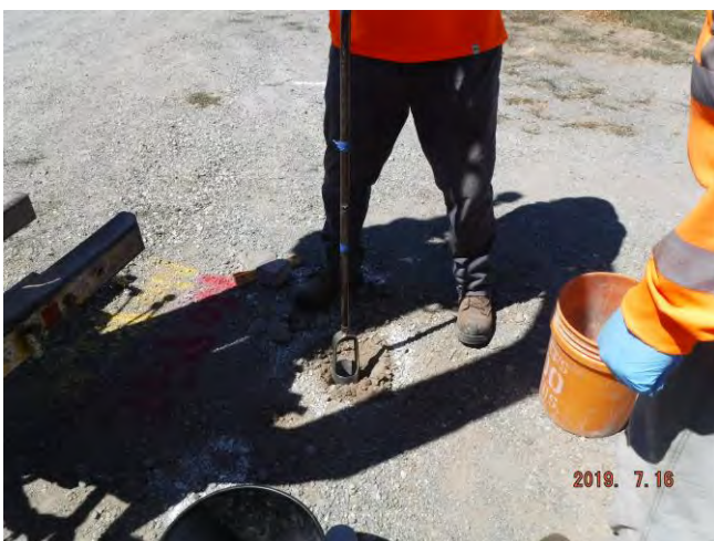
Photo 5: View of drilling boring B-8.
