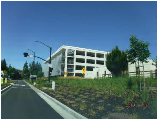
Photo 5: View of the Parking Garage, looking west.
