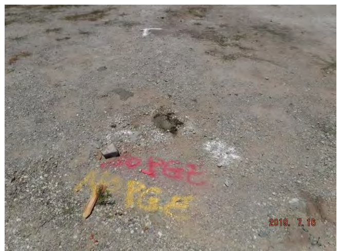
Photo 6: View of boring B-8 after drilling.
