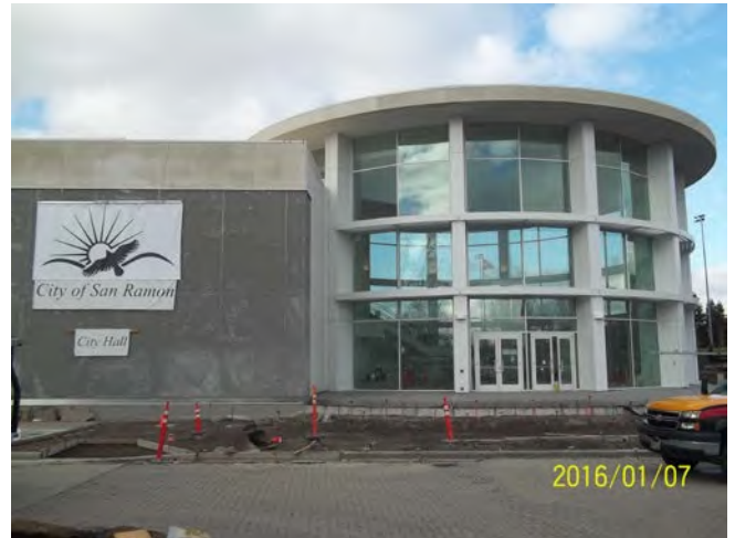
Photo 22: East – San Ramon City Hall, under construction (7000 Bollinger Canyon Road).
