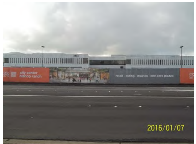
Photo 24: West – Camino Ramon followed by a commercial building, part of the San Ramon City Center Dev. Site.
