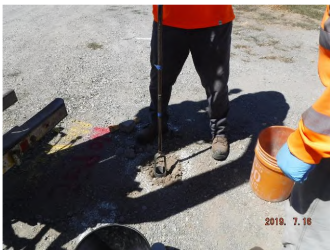
Photo 5: View of drilling boring B-8.
