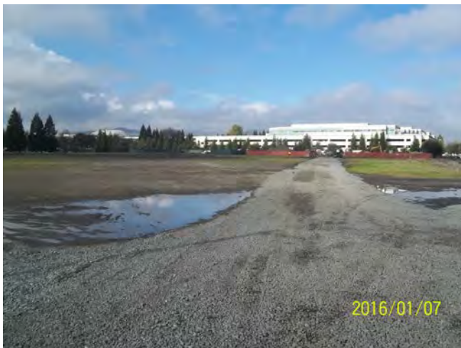
Photo 5: View of gravel access road, looking northwest.
