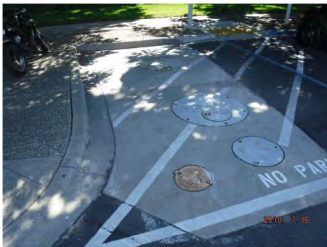
Photo 23: View of the north UST.
